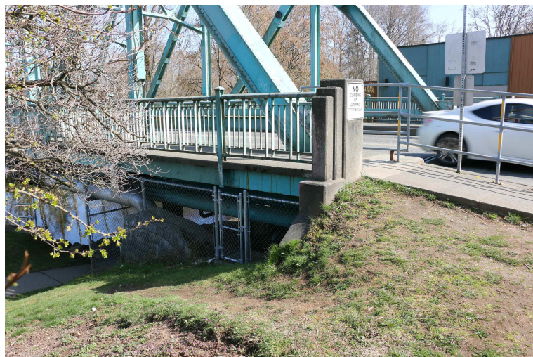
PHOTO SHOWING NORTH-WEST ABUTMENT, APRIL 3, 2018
