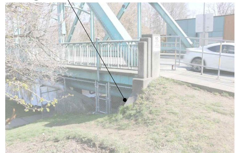
PHOTO SHOWING SOUTH-EAST ABUTMENT, APRIL 3, 2018
