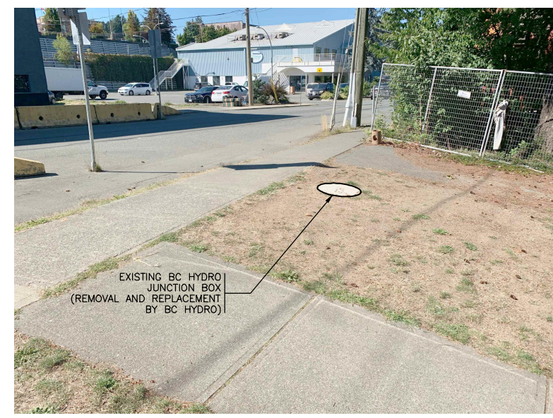
DETAIL E03 BC HYDRO JUNCTION BOX N.T.S.
